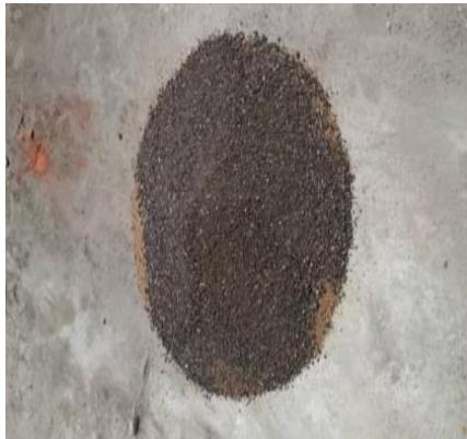
Fig.2. Mixing of concrete
