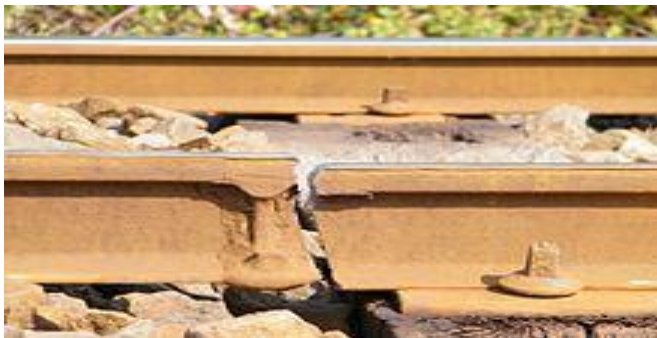
Fig (1) Crack on track
