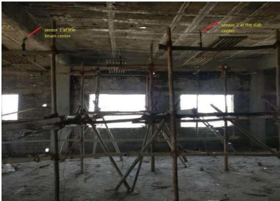
Fig.3. On-site picture of sensors location
