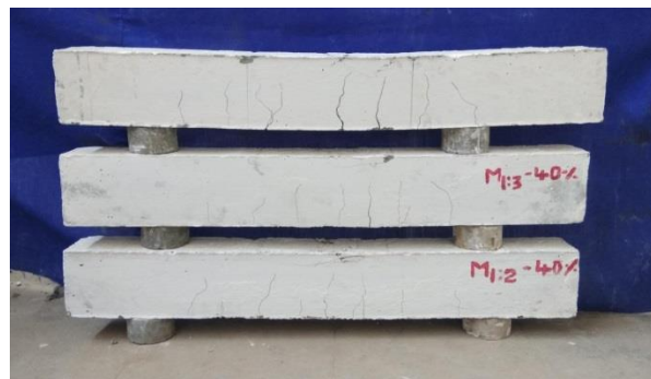
Fig.8. Tested beams of crack patterns
