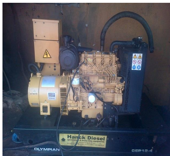
Figure 1.4 Completion of Corrective Maintenance.
